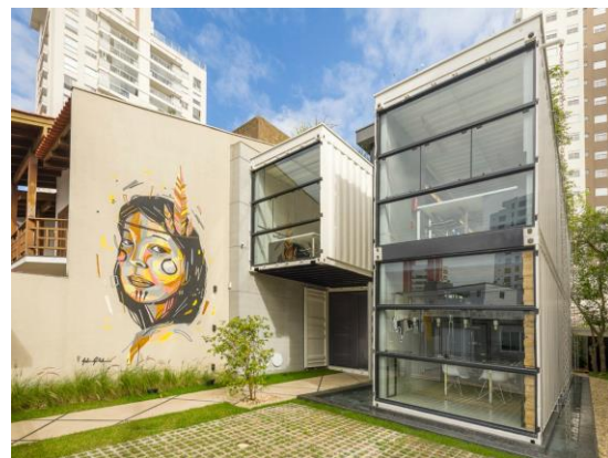
Gambar 4. Modular Building untuk Co-working Space di Brasil
