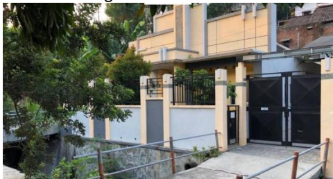
Figure 1. Front facade of a residential building in the Candisewu area, Semarang
