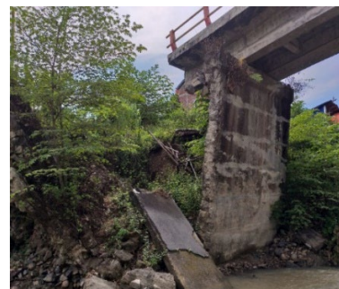
Gambar 16 Abutmen Roboh
