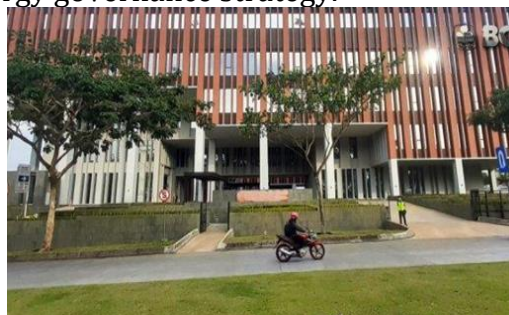
Figure 1. BCA of BSB Office Building
