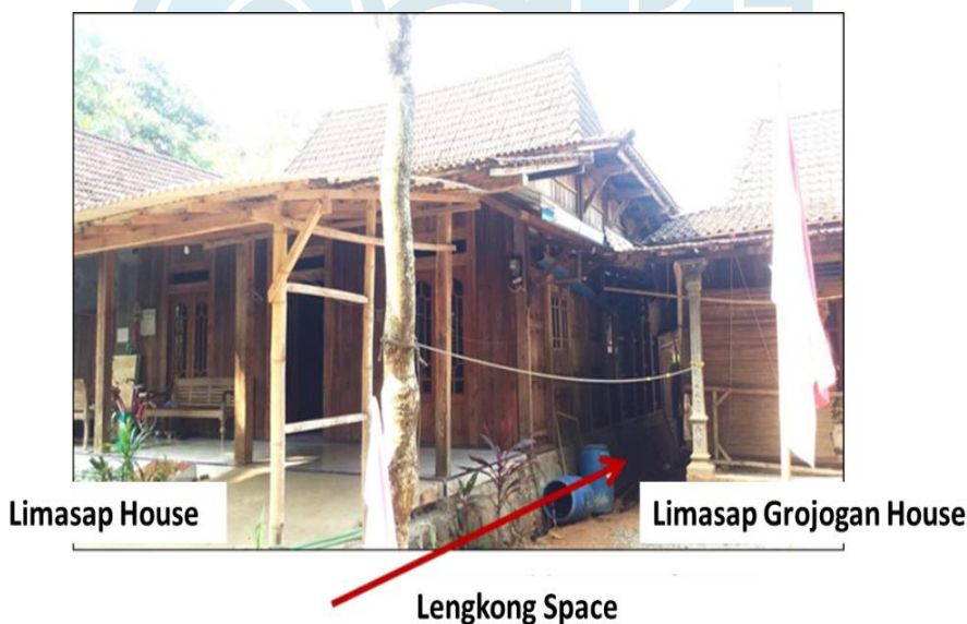
Figure 2: The Lengkong space between the Omah Limasap and Omah Limasap Grojogan (Setiohastorahmanto, 2023)
