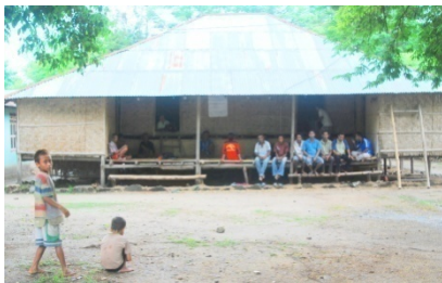
Picture 1: a “traditional” house
