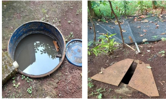
Figure 2. The First Tank, Second Tank, And Final Reservoir
